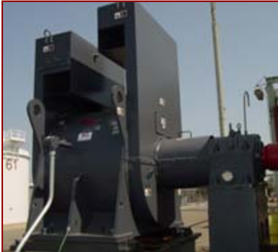
Complete Exciter with Enclosure (located at Philips 66 in California. Attached to GE Motor)
