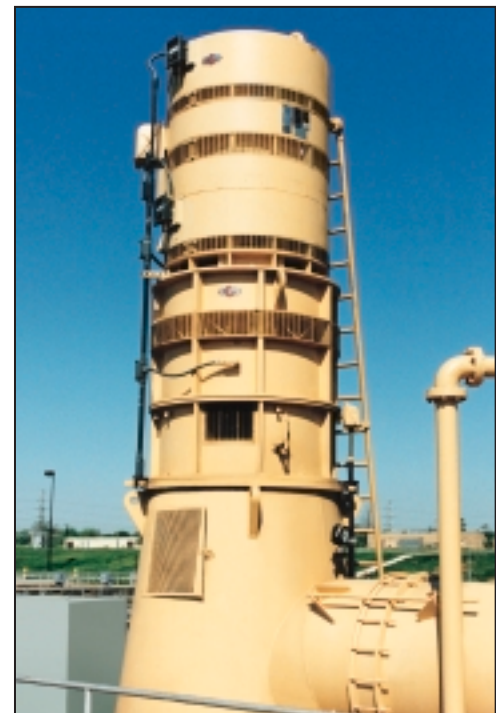
Vertical drive with EM Induction Motor.
